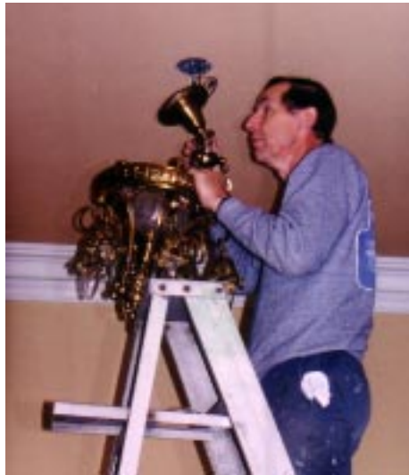
Bob Carey installing teardrop chandelier in the dining area.
