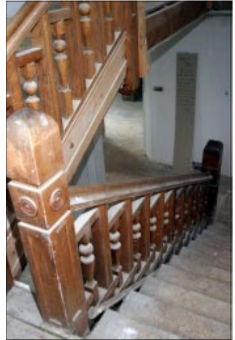
The bannister—many hours of restoration.
